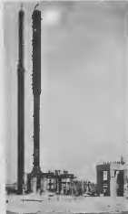
On left picture, HDS Instructors M. Leo (left) and B. Alders pose with model of HDS Hydrogen plants. On right picture, two towers, the CO2 absorber (left) and the Catacarb Regenerator, are now installed at Hydrogen Plant No. 1.
